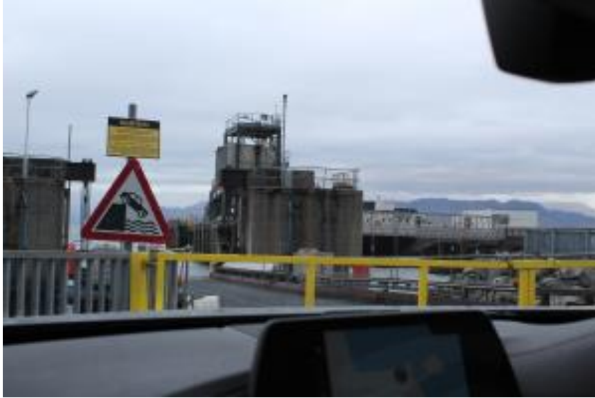
Ferry Terminal Armadale
