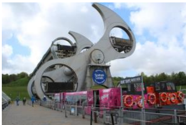
Falkirk Wheel slowly lowering
