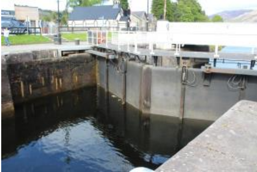
Caledonian Canal lock section
